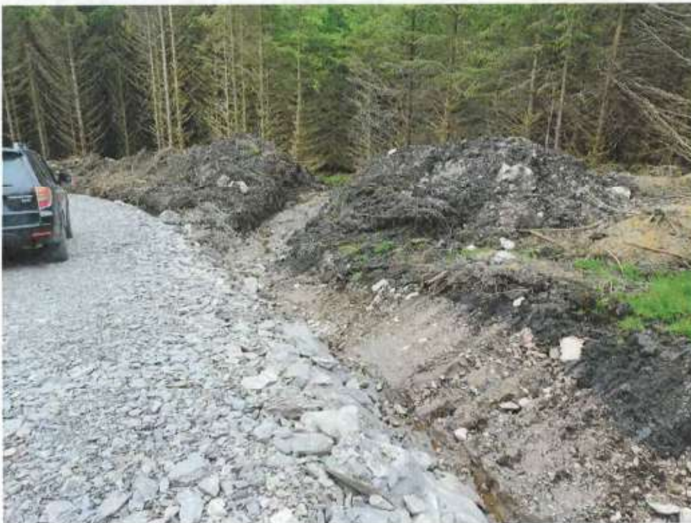
New access track and drainage associated with ongoing forestry activities observed during site surveys 16/06/2020.
