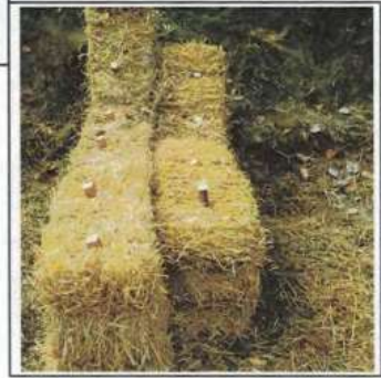
Example of a Strawbale Checked Dam (Kawartha Conservation, 2020)
