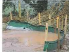
Example of Silt fencing in use [EnviroPro, 2022] Available at: < https://www.enviropro.co.uk/entry/153977/Siltbuster/Terrastop-silt-fences-for-erosion-and-runoff-control/ >
