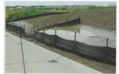
Example of Silt fencing in use Bowman Construction Supply (2023) Available at: < https://www.bowmanconstructionssupply.com/products/silt-fence/ >
